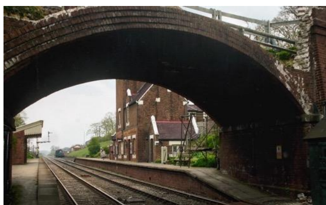
North Rode Railway Station Bridge
