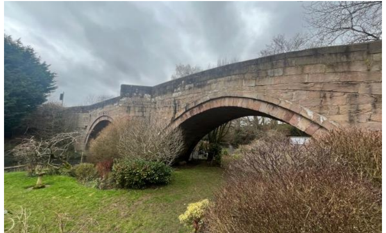
Colley Mill Bridge
