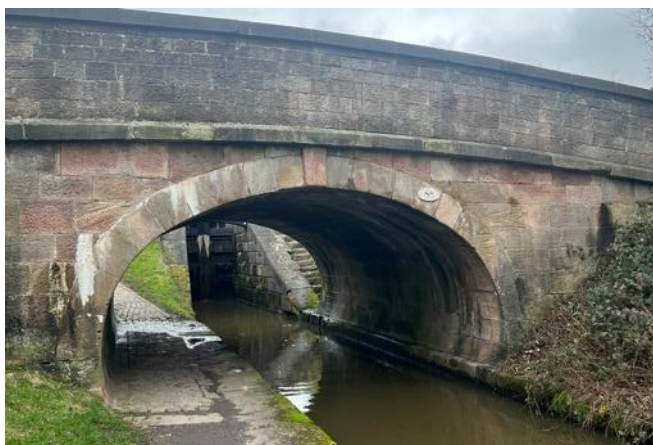
Macclesfield Canal Bridge 55
