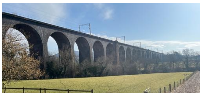
North Rode Viaduct
